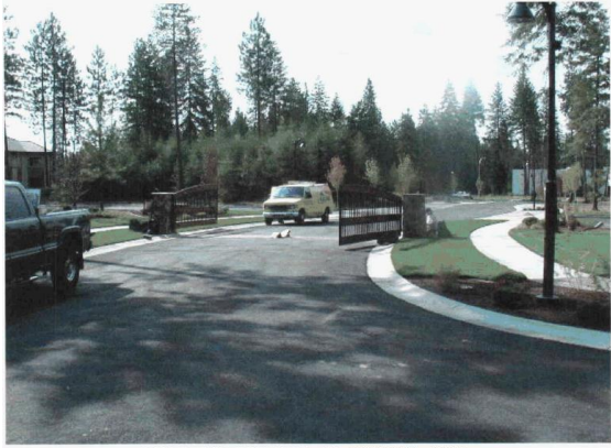
GATE BETWEEN RESIDENTIAL AND COMMERCIAL AREAS
