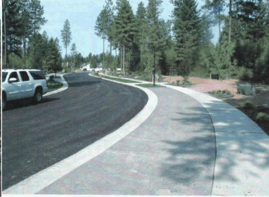
STAMPED CONCRETE ROADSIDE PARKING AREA
