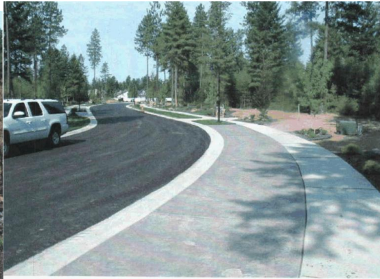
STAMPED CONCRETE ROADSIDE PARKING AREA
