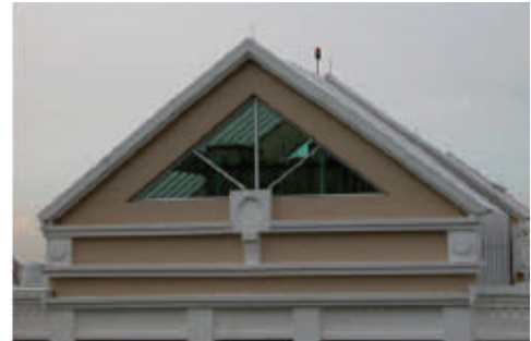
enclosed mechanical rooftop equipment
