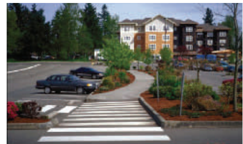
pedestrian path through parking lot
