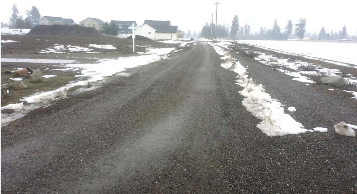
Alps looking east (Emergency Fire access for Phase 2):
