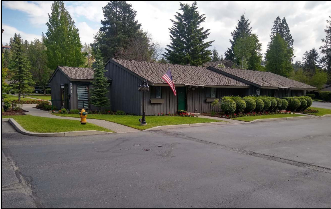
SITE PHOTO 2: View from Sherman Avenue looking north toward office building.
