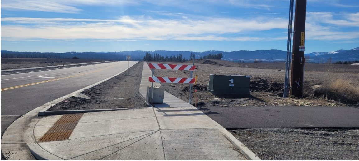
Intersection of Hanley Ave. & Alecat Dr. looking southwest into 14-acre rezone request:
