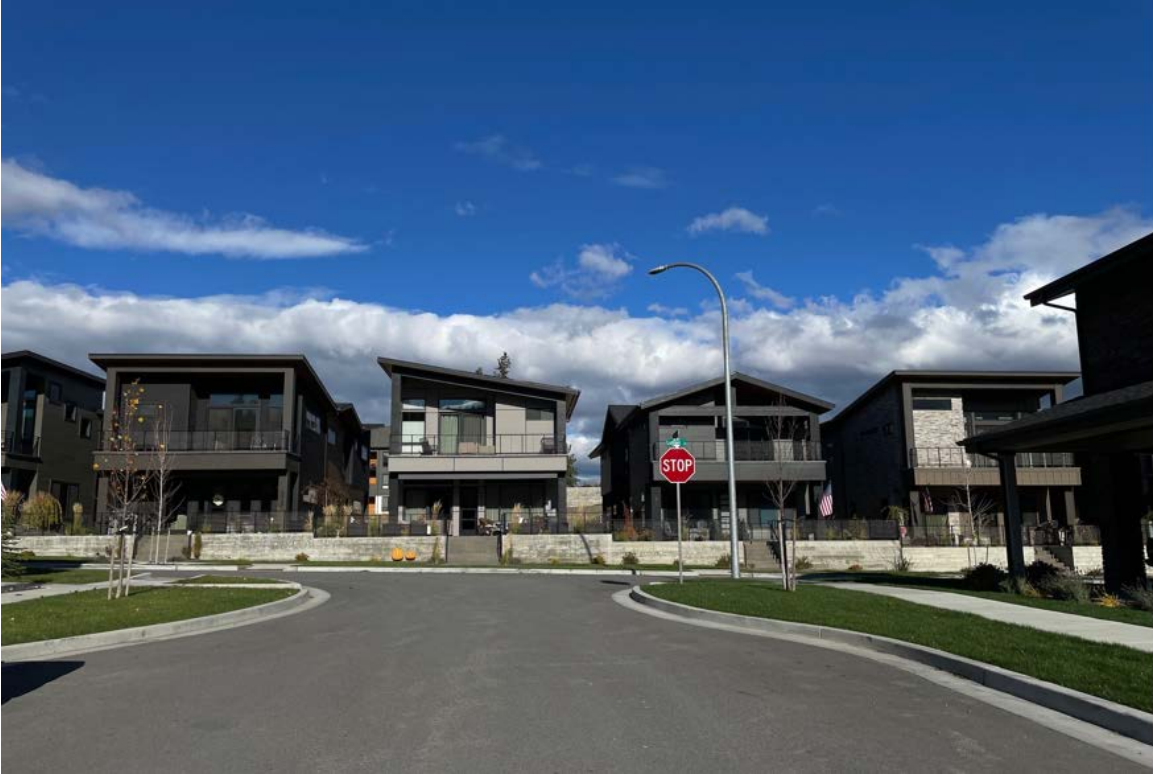
SITE PHOTO 6: Development Area 8 south of the alley looking north from Kiln Road (houses fronting Lumber Lane)
