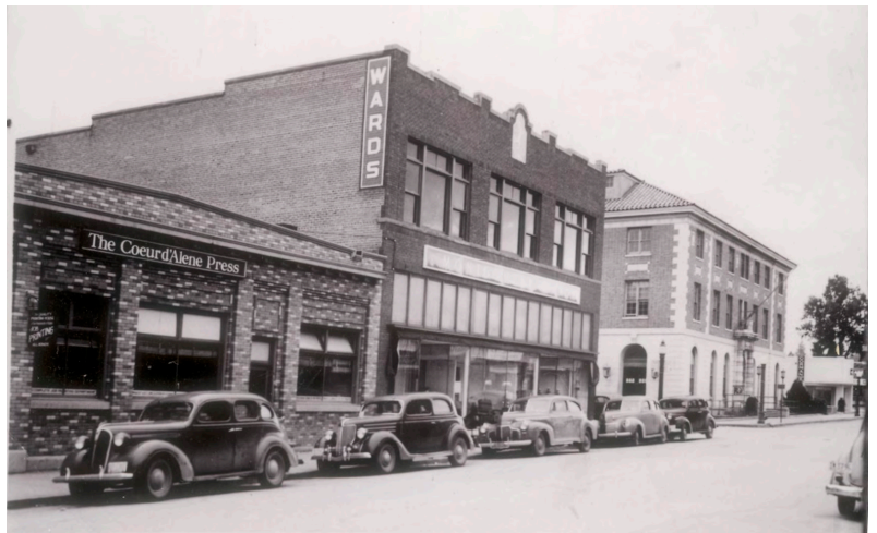
Figure 24. The Coeur d’Alene Press building and the Montgomery Ward building The Coeur d’Alene Press building is a one-part block and the Montgomery Ward building is a two-part block. Courtesy City of Coeur d’Alene.
