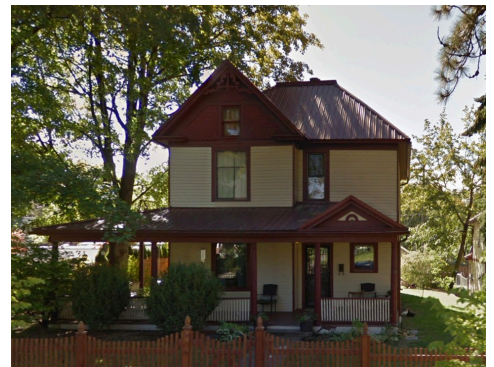
Figure 34. 712 E Foster Avenue
