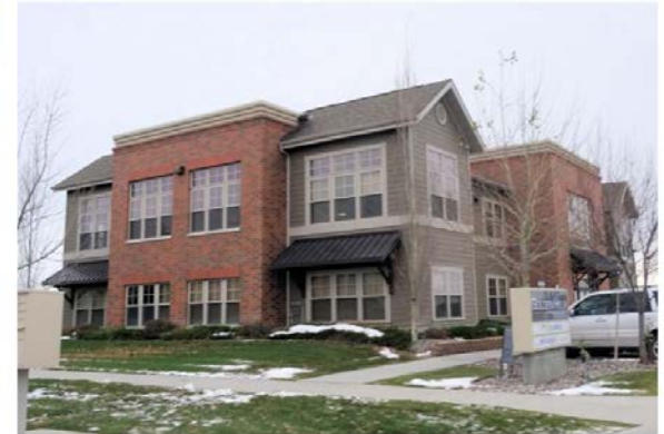
The left building illustrates a pitched roof example and the right building includes a combination of flat and gabled rooflines.
