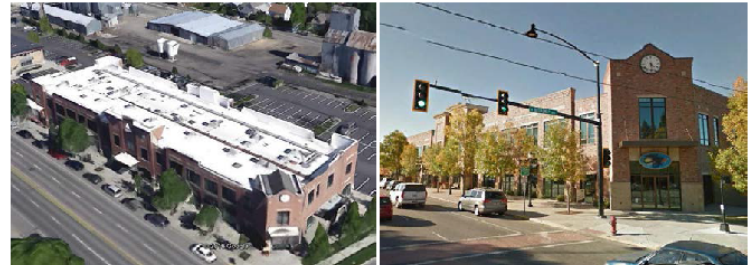
The top illustration and the East Main Street building aerial and street view illustrate examples of rooftop mechanical equipment that has been screened by walls (top illustration) or parapets (East Main Street building).
