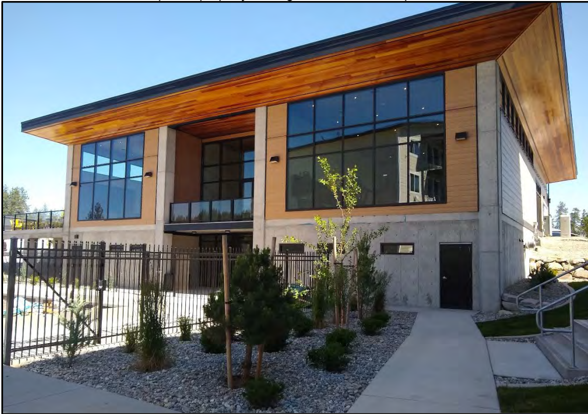
SITE PHOTO - 3: Central part of property looking north toward the apartment's clubhouse.
