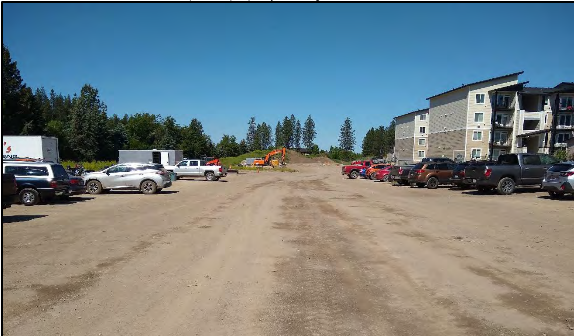
SITE PHOTO - 5: South central part of property looking west.
