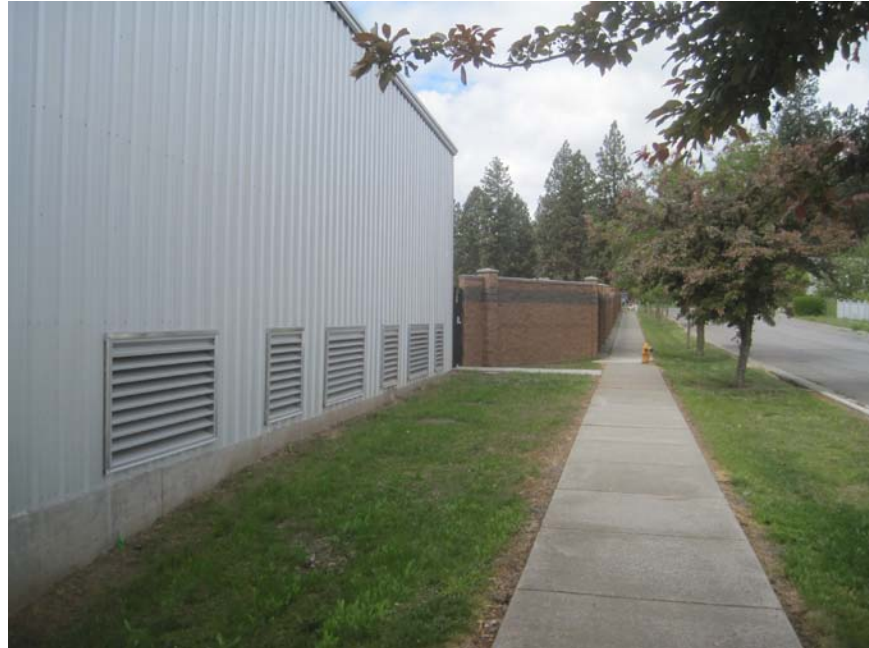
Photo 5. Wall mounted louvers on the north side of Doyle's Warehouse.
