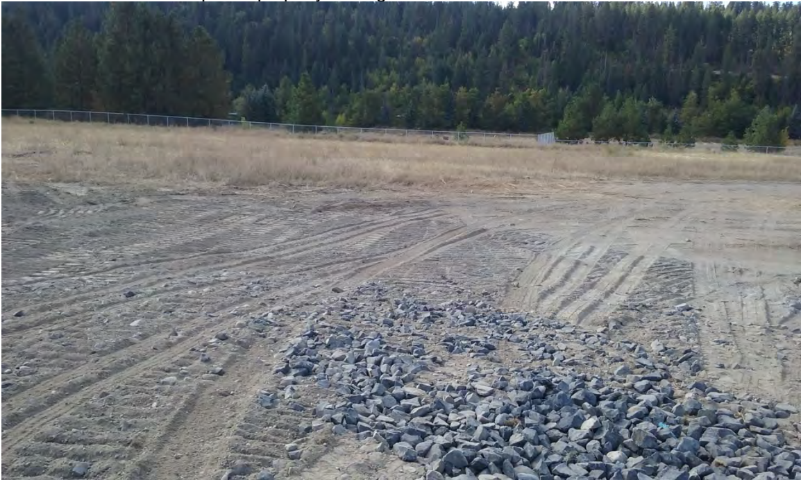
SITE PHOTO - 5: North part of property looking south.
