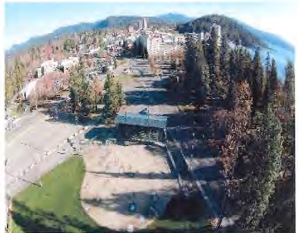
Figure 6 Mullan Road/Government Way & Northwest Boulevard Create the "Four Corners".
