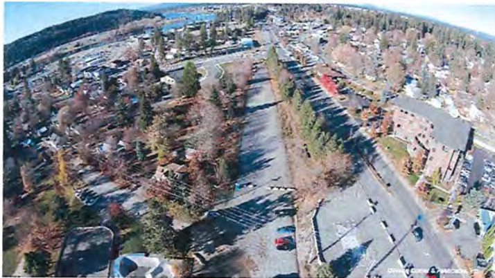
South end of BLM Corridor Looking North
