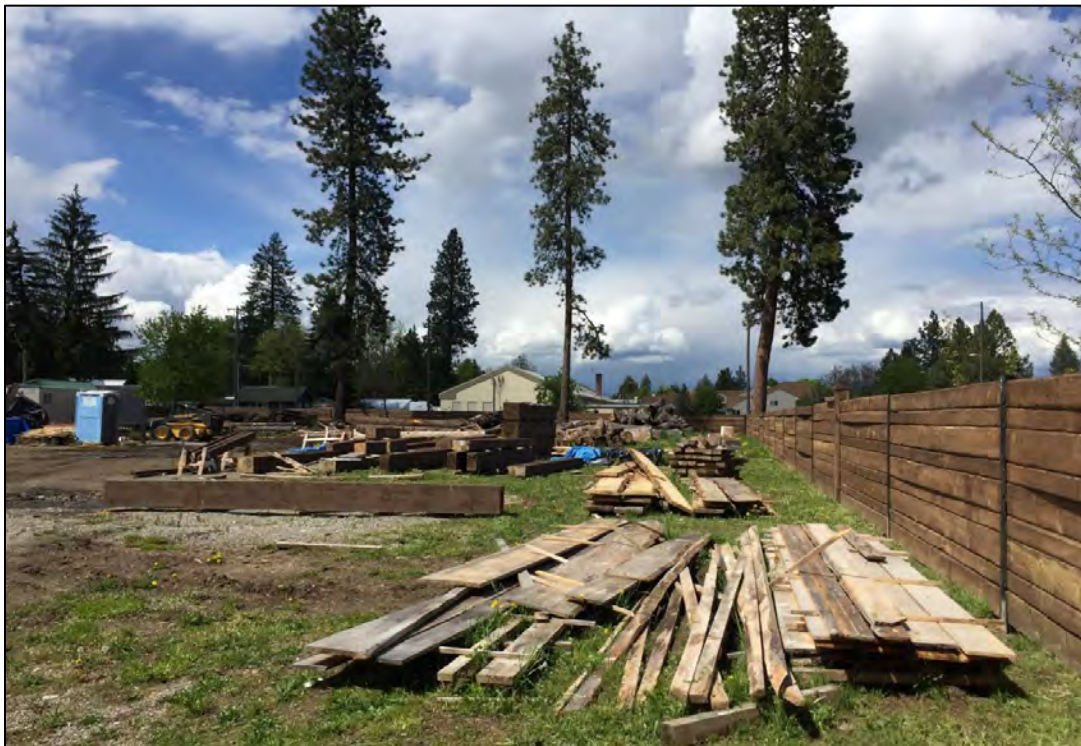
View of the subject property from Spokane Avenue looking north toward the NIC Armory Building.
