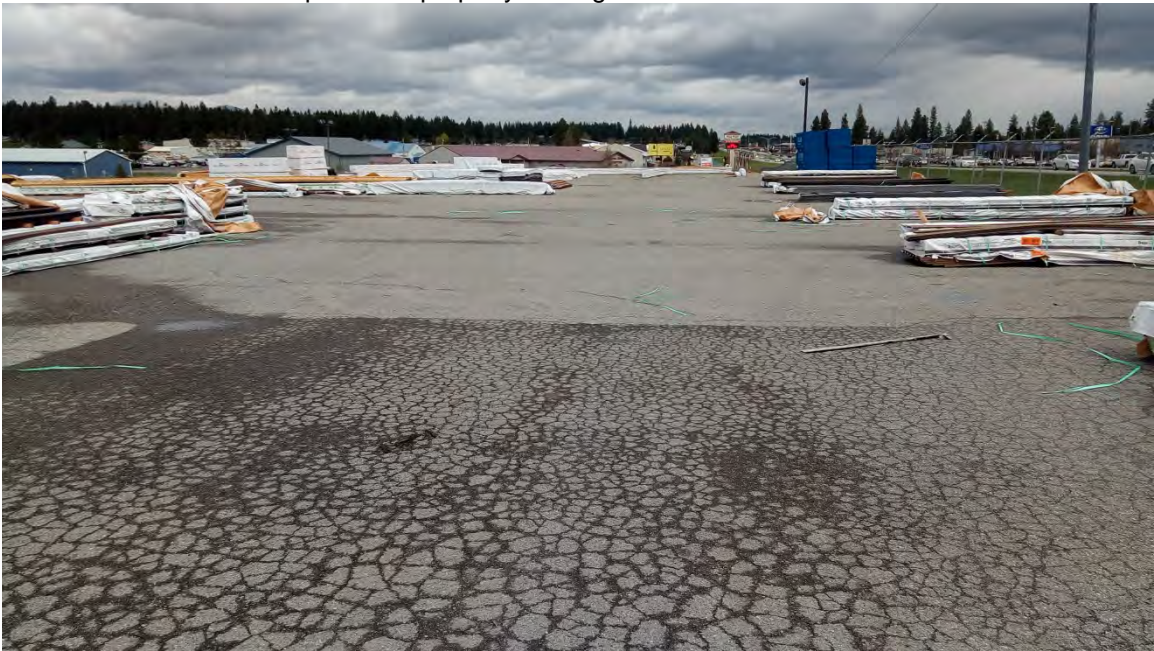
SITE PHOTO - 2: Center portion of property looking south.
