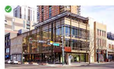
Current era construction, floor to floor heights, color, tripartite.
