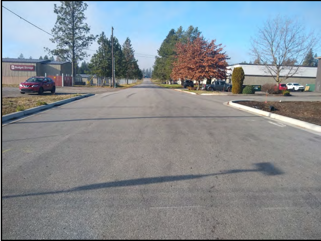
SITE PHOTO - 4: View from the intersection of Government Way and Aqua Avenue looking east.
