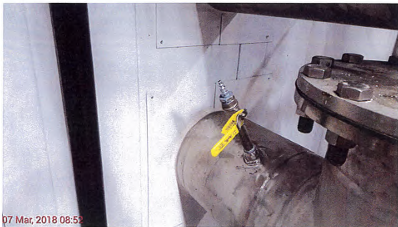
Photo 1. Finished air piping used for start-up/future bubble testing for leaking cassettes/filter strands. Piping is attached using a 1/2" weld-o-let.
