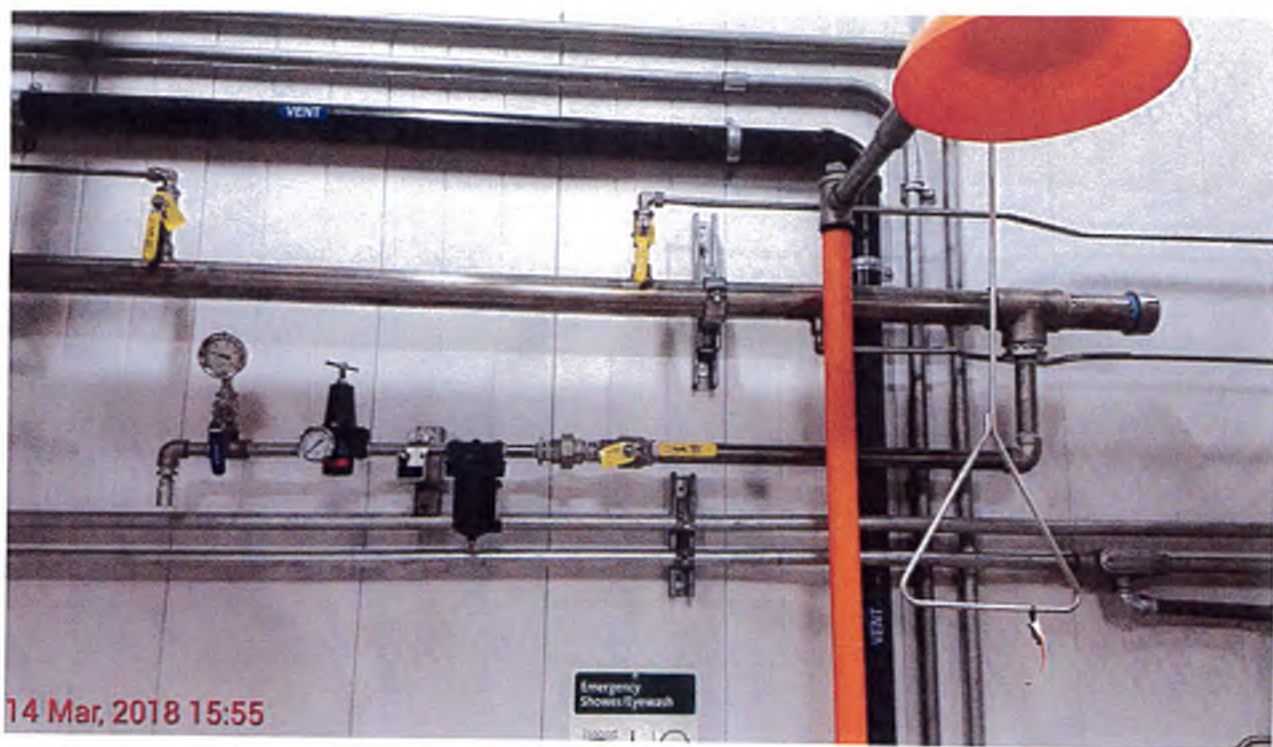
Photo 2. Finished air supply manifold.
