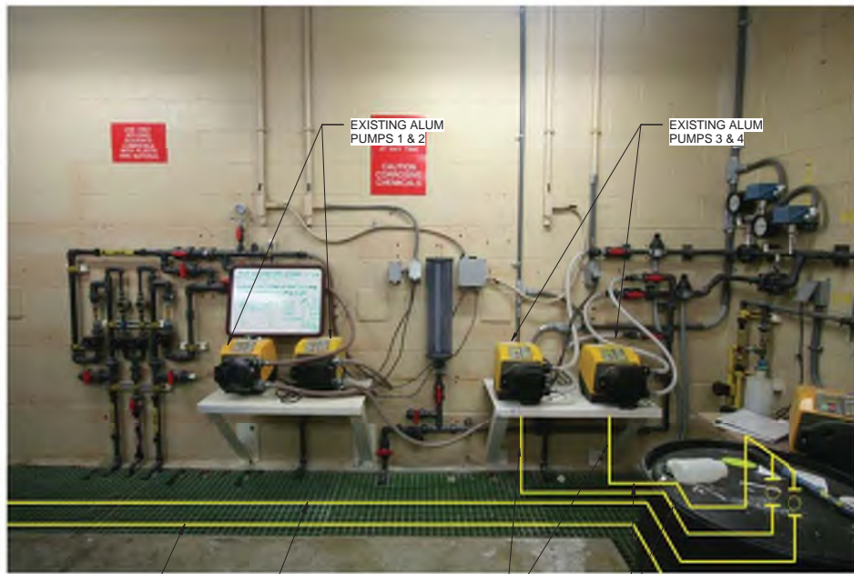
1 ALUM PUMP PHOTO 1 570D101 NOT TO SCALE
