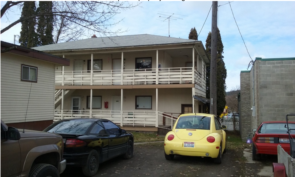
SITE PHOTO - 4: View from the center part of property looking west.
