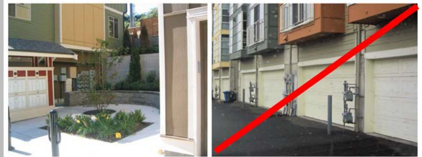
Place utility meters in less visible locations. The upper and lower left examples are successfully tucked away in a less visible location and/or screened by vegetation. The right images are poorly executed and would not be permitted in such visible locations. Such meters must be coordinated and better integrated with the architecture of the building.
