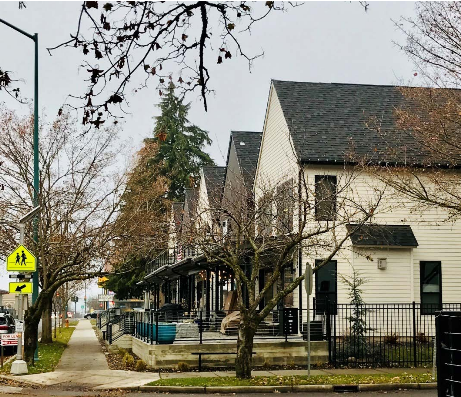
Current Example of Coeur Housing on East Sherman Avenue.
