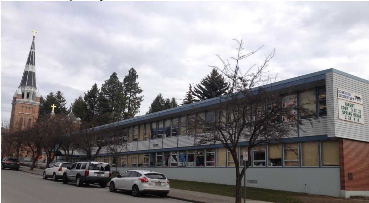
Sorensen Elementary- looking northeast
