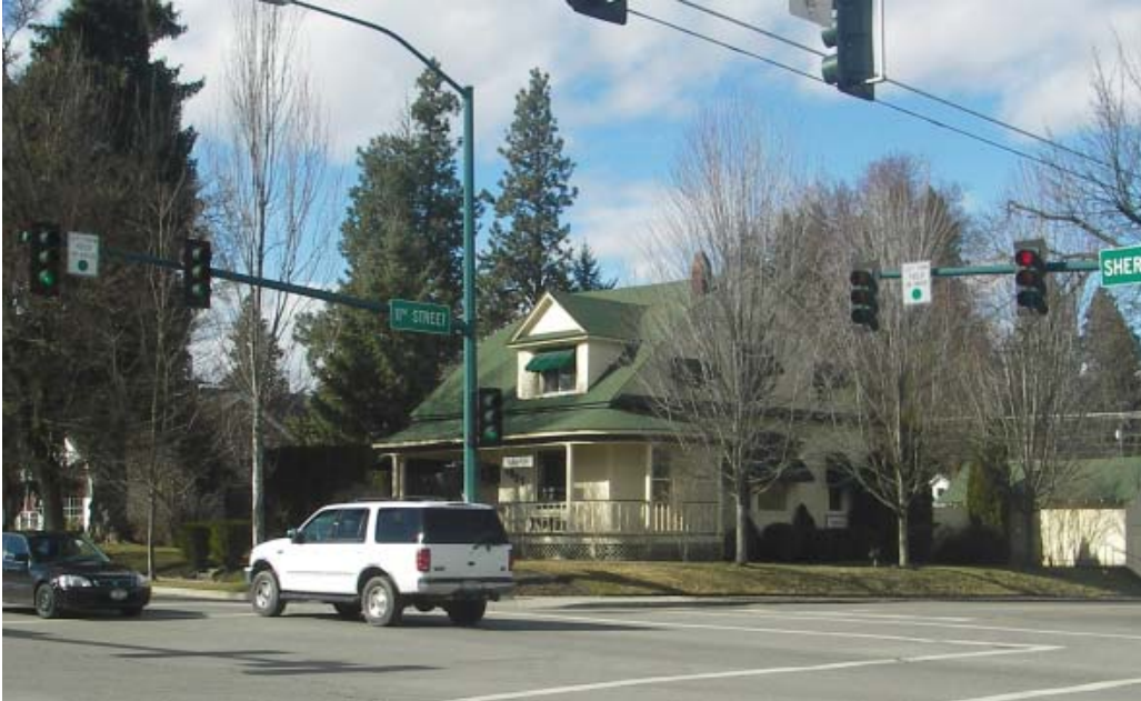
G. Existing building on subject property
