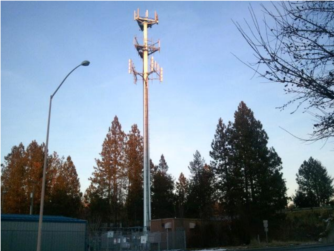
Existing Wireless Tower site near 24 th & Sherman Ave:
