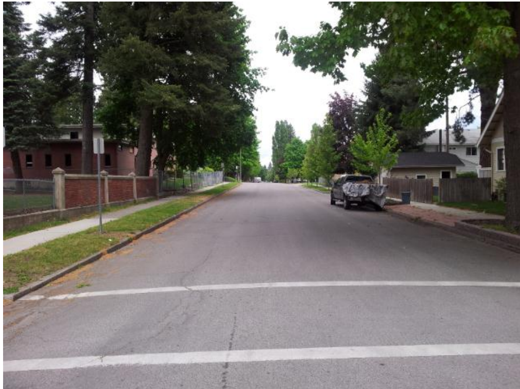
10 th Street from Coeur d'Alene Ave. (Facing North)
