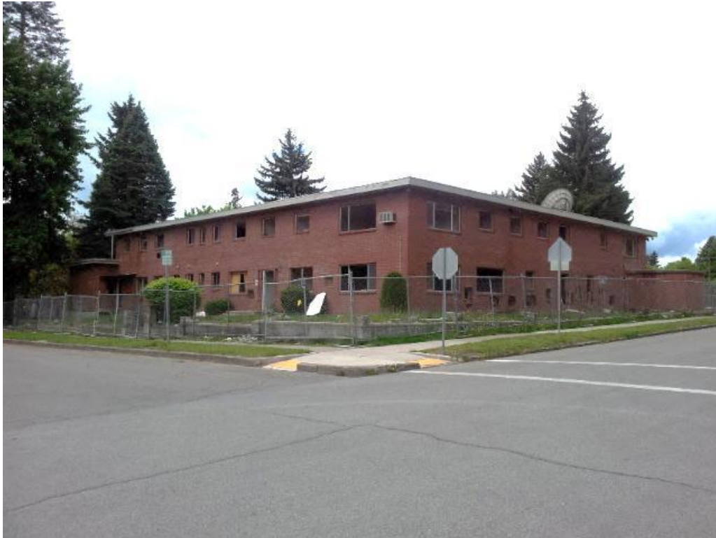
Administration building from Indiana and 10 th (Looking SW)
