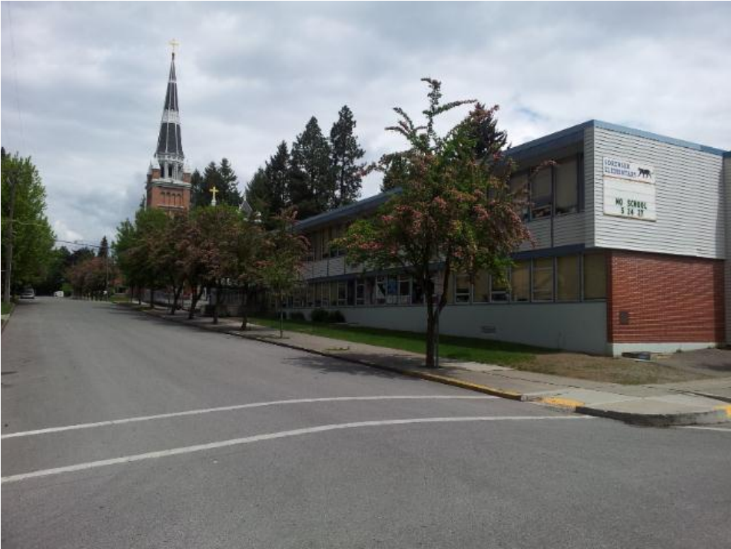
Sorensen Elementary from intersection of Coeur d'Alene Ave & 9thSt.
