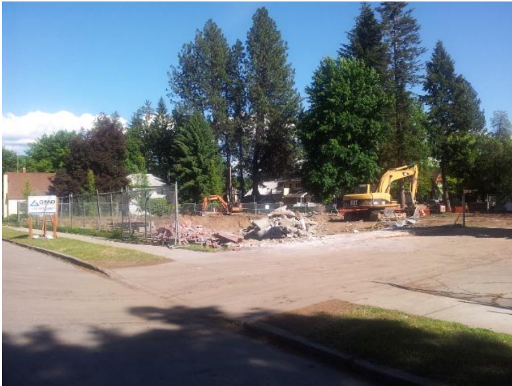
Removed administration building from Indiana (Looking SE)
