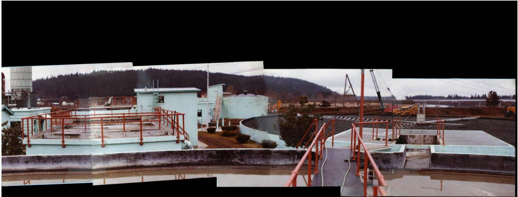
View from top of Primary Clarifier
