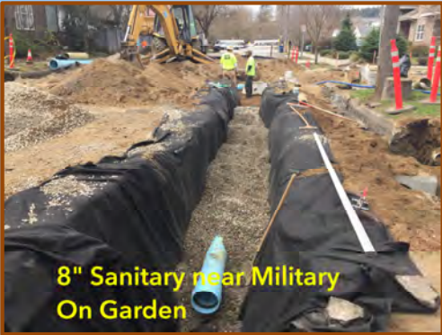
Open Trench Replacement
