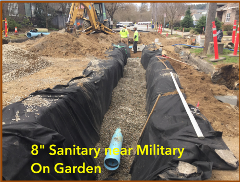
Open Trench Replacement
