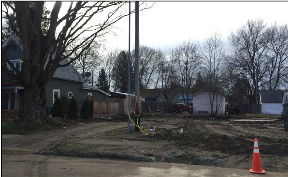
View of the 4 th Street Lofts from Reid Avenue looking south toward future parking area
