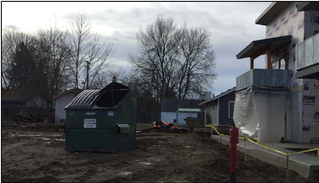
View of the 4 th Street Lofts from Reid Avenue looking south toward future parking area
