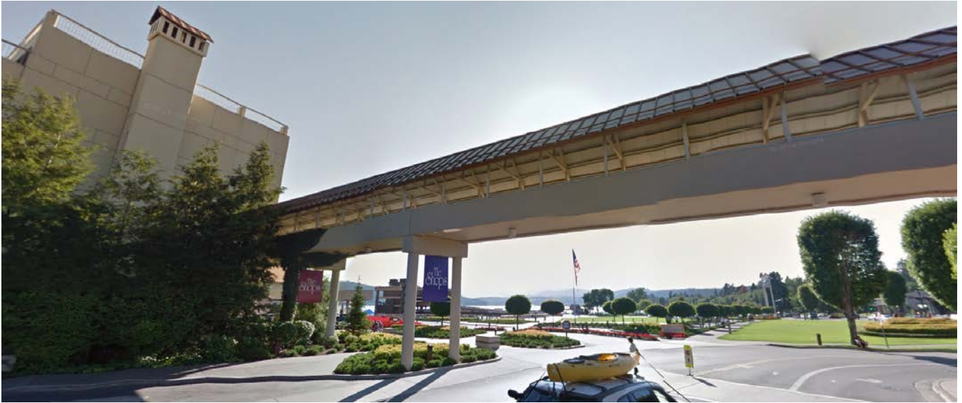
SITE PHOTO: LOOKING WEST TOWARD SUBJECT PROPERTY:
