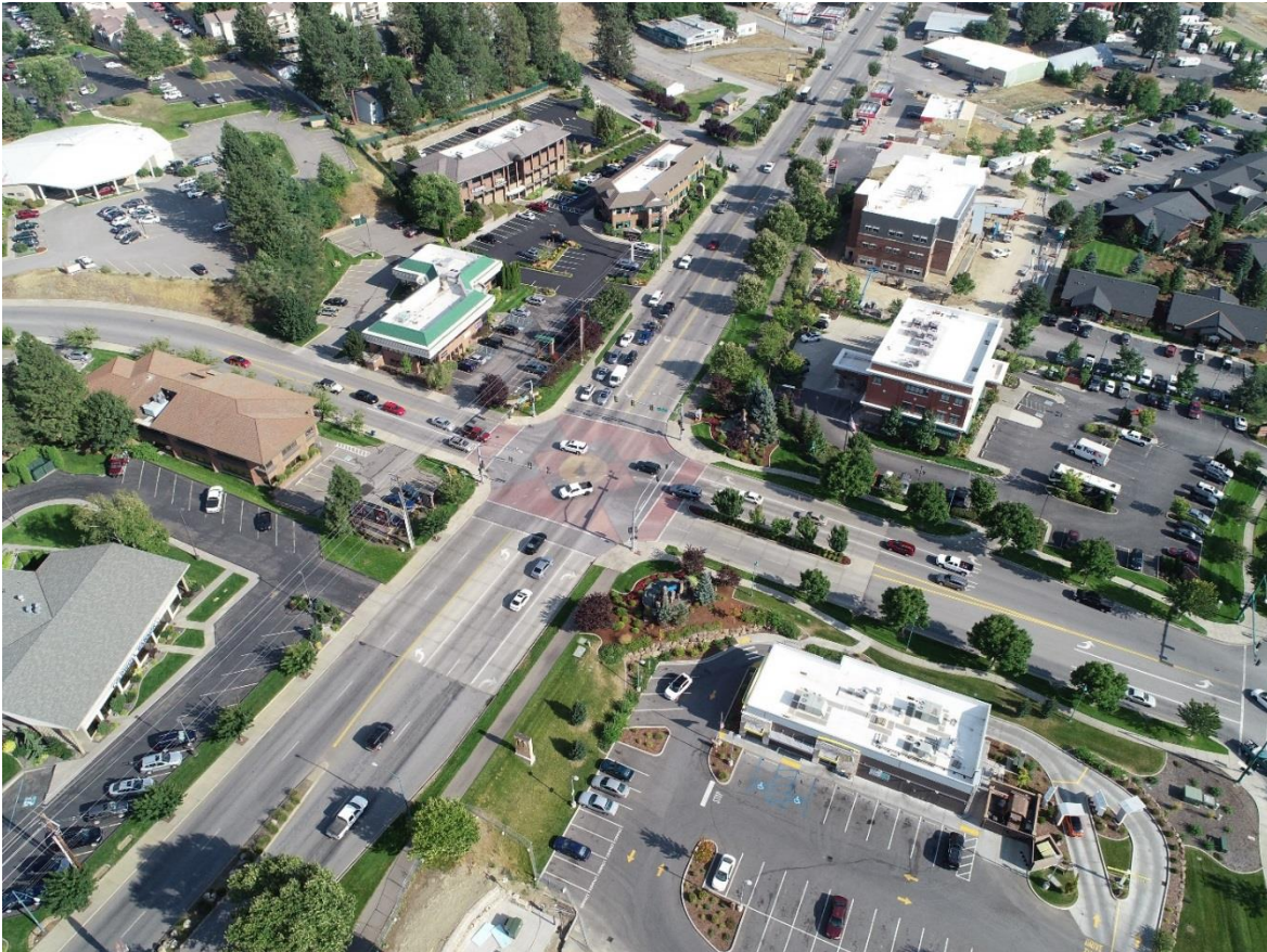
Figure 10-2: Intersection of Lakewood & Northwest Boulevard
