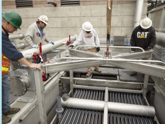
GE Membrane Filter Cassette Being Installed in Membrane Tank
