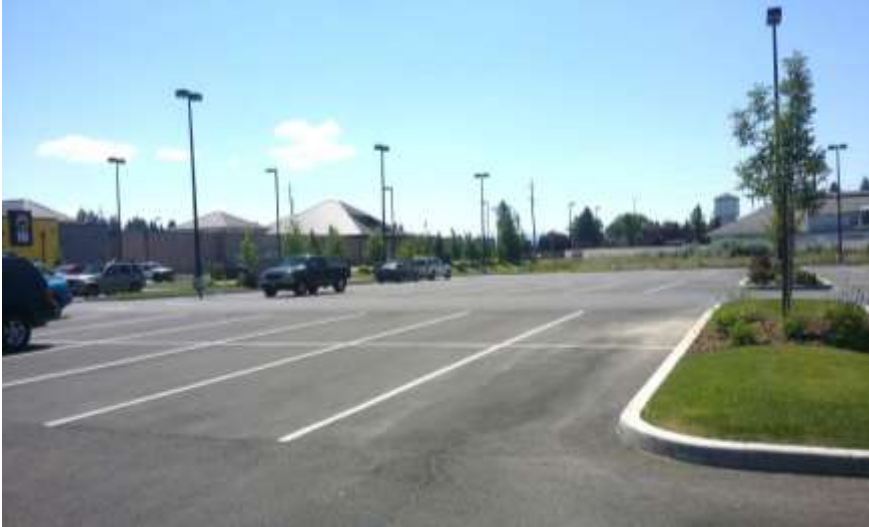
Developed parking lot looking southwest toward Neider Ave.:
