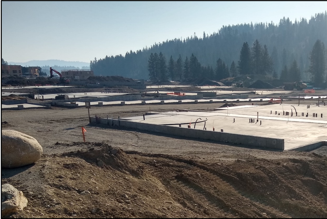
SITE PHOTO - 5: North central part of property looking southeast.
