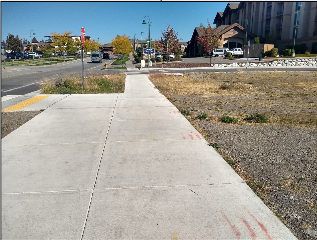
SITE PHOTO - 2: View from Beebe Blvd looking northeast
