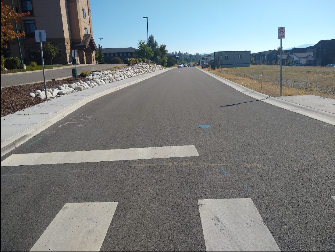
SITE PHOTO - 3: View from the intersection of Beebe Blvd and Union Drive looking southeast.
