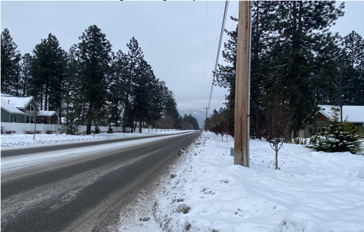
SITE PHOTO - 4: View looking east along Hanley Avenue:
