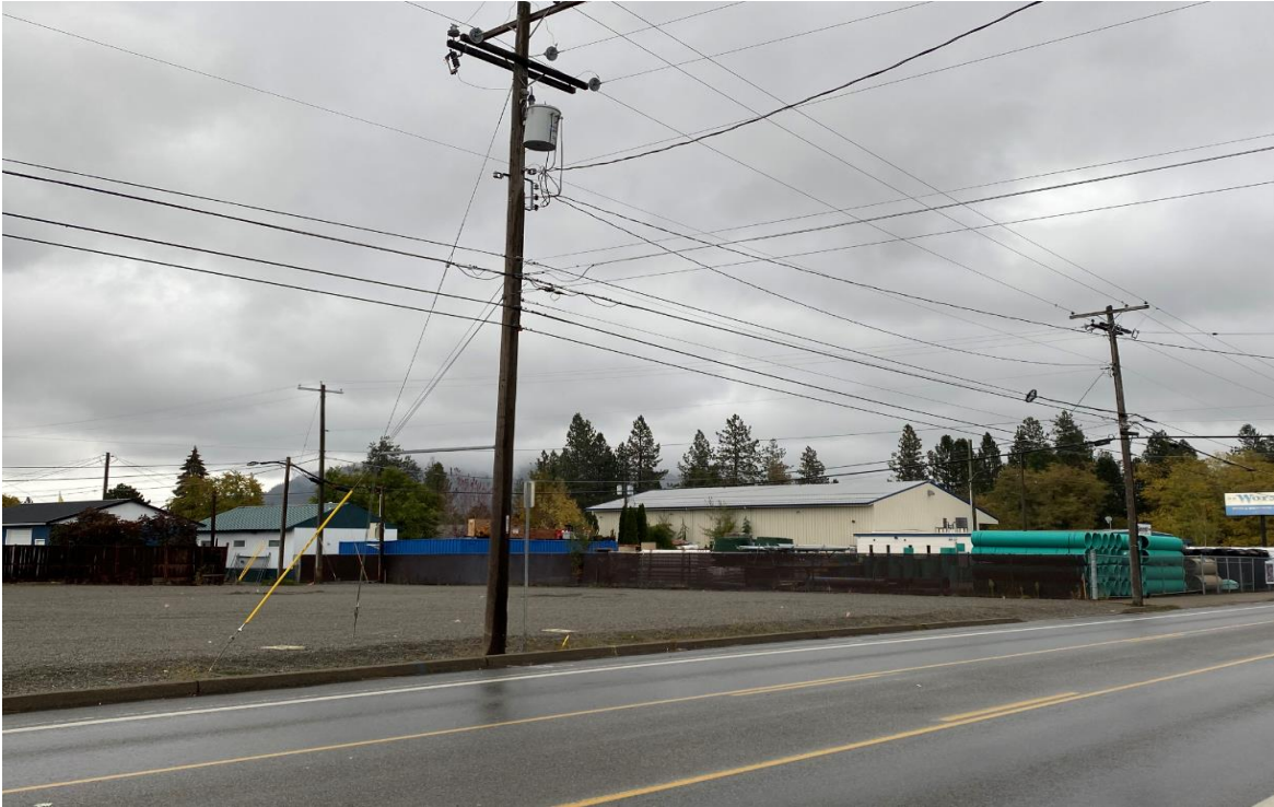
Looking northeast at the subject property from Best Avenue (comprised of 3 lots)
