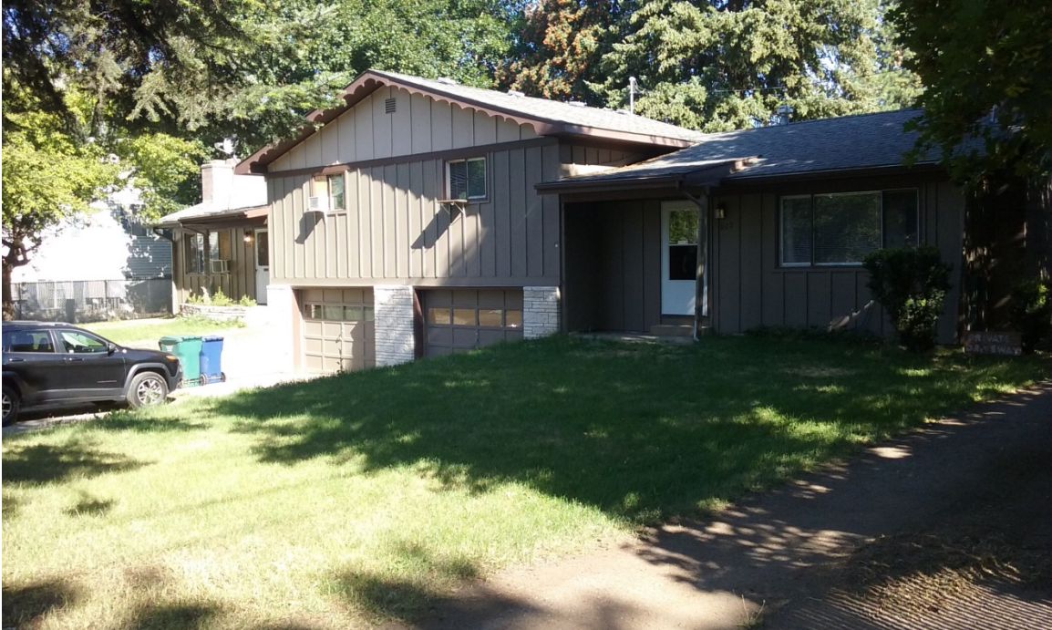
SITE PHOTO - 1: Southeast part of property looking northwest.
