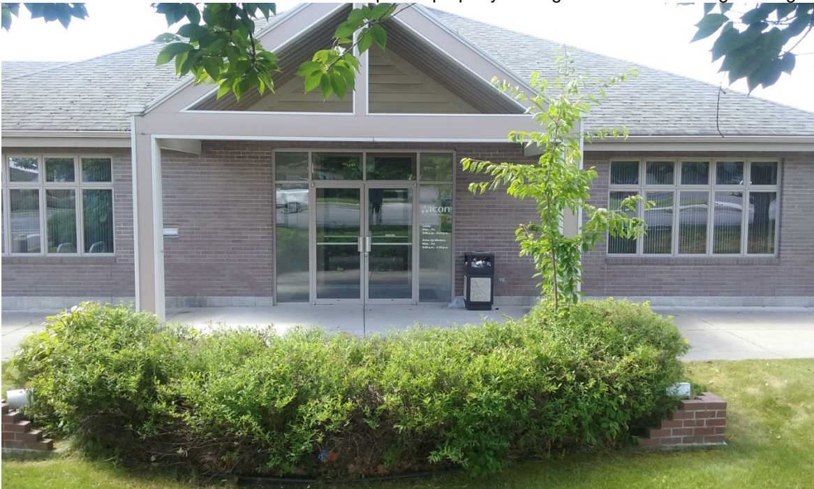
SITE PHOTO - 3: View from the north central part of property looking south at the existing building.
