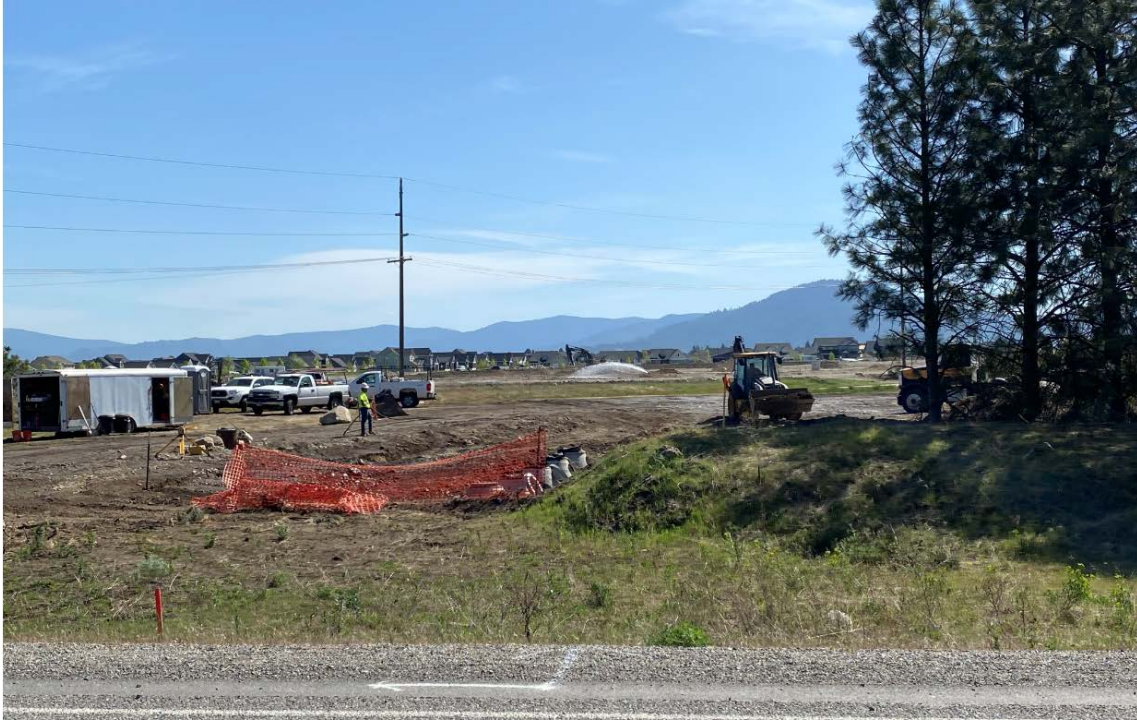
SITE PHOTO - 3: Looking east at the subject property from Huetter Road.
