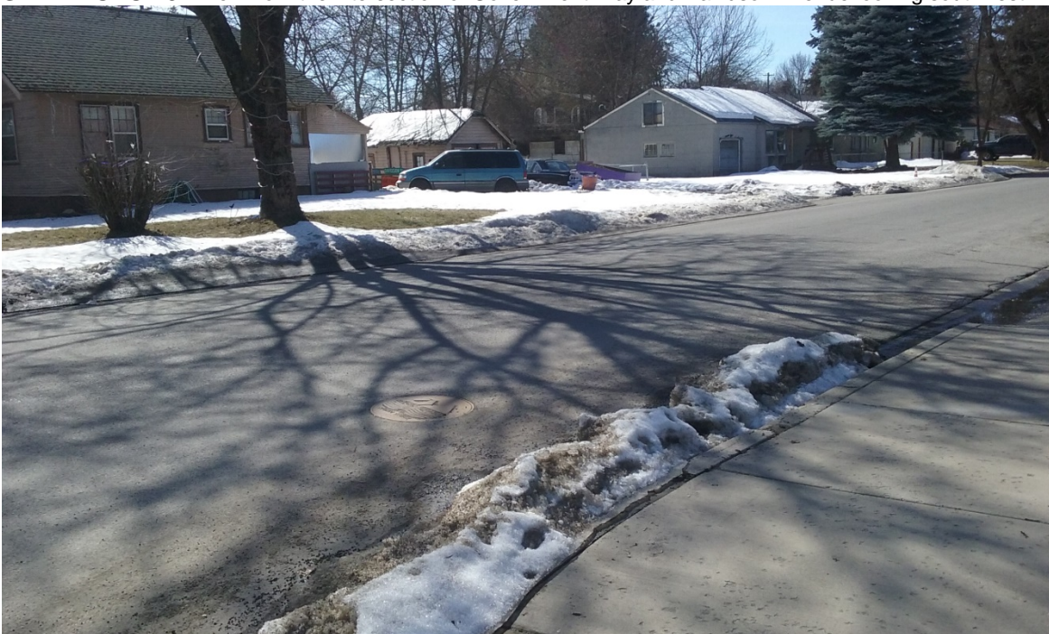
SITE PHOTO - 5: View from the intersection of Government Way and Davidson Avenue looking southwest.
