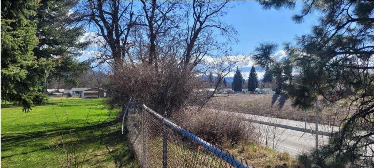
State ROW fencing looking east showing grade change to I-90 (4 th Street exit below):
