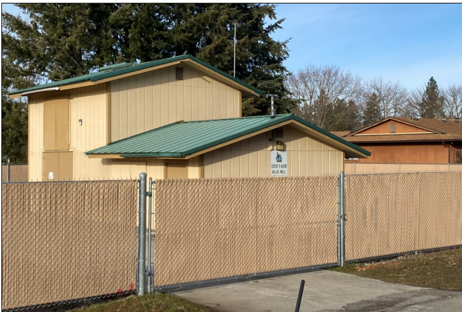
View looking northwest along Atlas Road at the well house.
