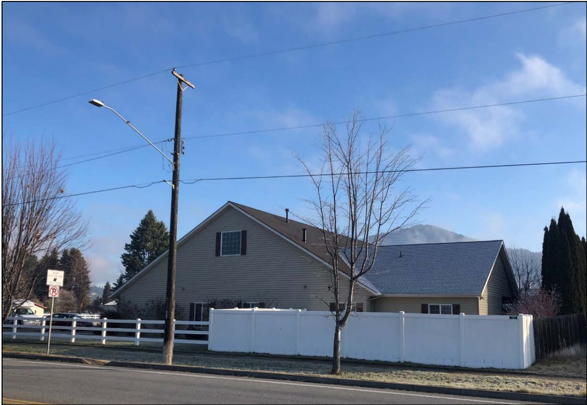
SITE PHOTO- 4: View along 4 th Street looking east toward the subject property at one of the residential care buildings
