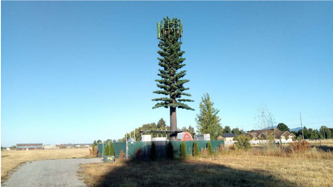
Stealth cell phone tower onsite (Verizon) looking west showing gravel access:
