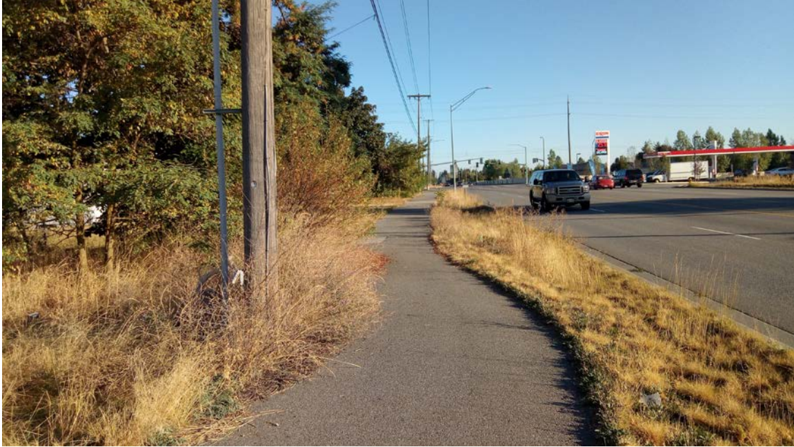
Ramsey Road looking north toward Prairie Avenue showing asphalt trail :
