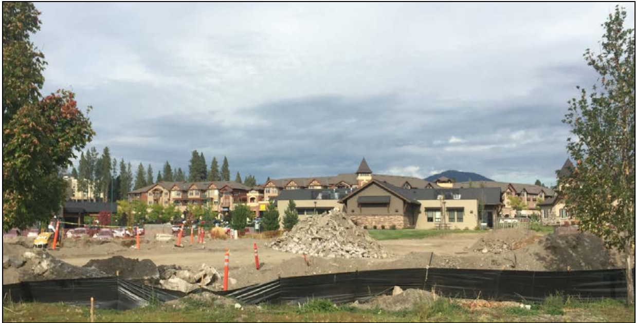
SITE PHOTO - 6: View from the southeast corner of property looking north toward the Pain Management of North Idaho building.
