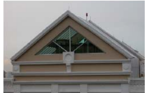
enclosed mechanical rooftop equipment
