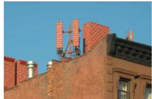
cell transmission equipment integrated into brick building
