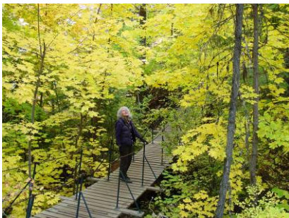
Tubbs Hill Suspension Bridge
