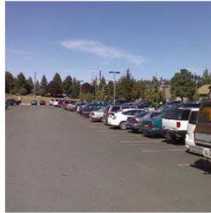
Existing development patterns are suburban, with a heavy reliance on surface parking.
