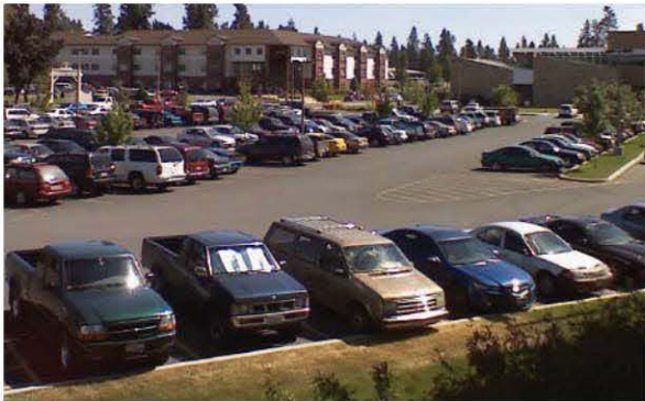
The traditional development pattern on the campuses has been defined by large, stand-alone buildings and large surface parking lots.
