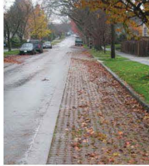
An example of pervious pavers in the parking lane to facilitate stormwater infiltration.
