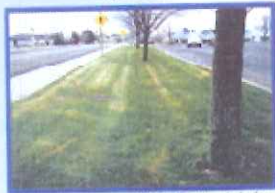
Grassy swales provide bio-filtration to help prevent pollutants in street runoff from getting into the groundwater.
