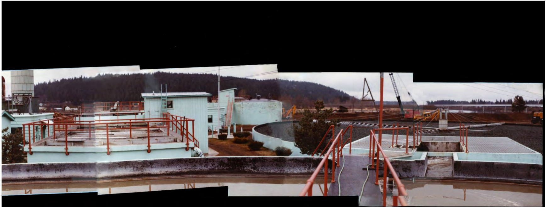
View from top of Primary Clarifier
