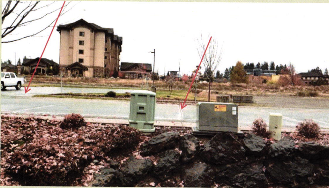
Looking north towards the Centennial Trail
